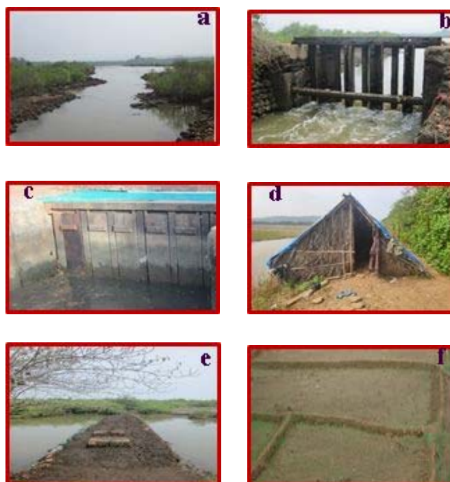
Figure 2. Structure of khazan ecosystem, (a) Water canal (b) Sluice gate (open) (c) Sluice gate (closed) (d) Hut near manos (e) Outer embankment (bandh) (f) Inner embankment (mero)
