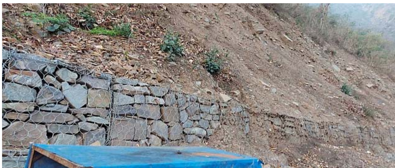
Figure 7. Anti-erosion work, Rudraprayag
