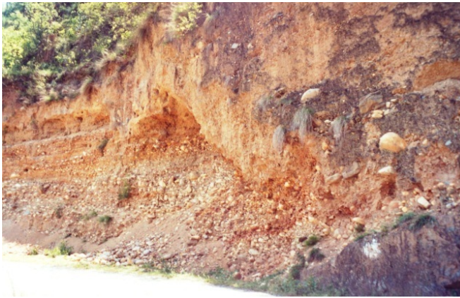
A. Erosion due to landslides
